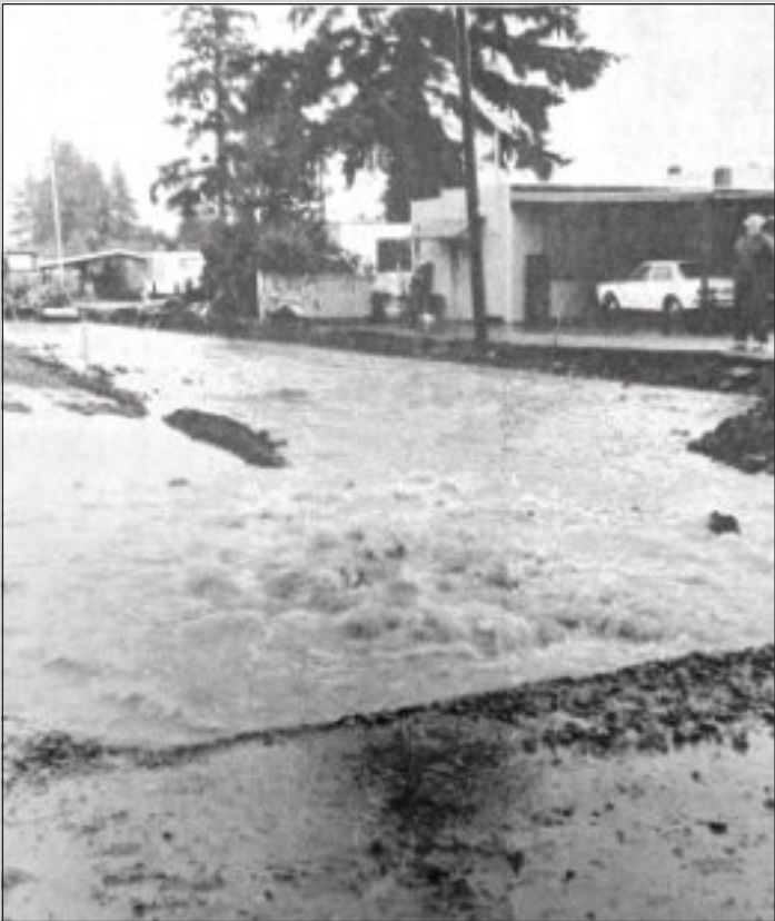
A pond formed on 15th Avenue after excavation disturbed a water line stub in 1975.
