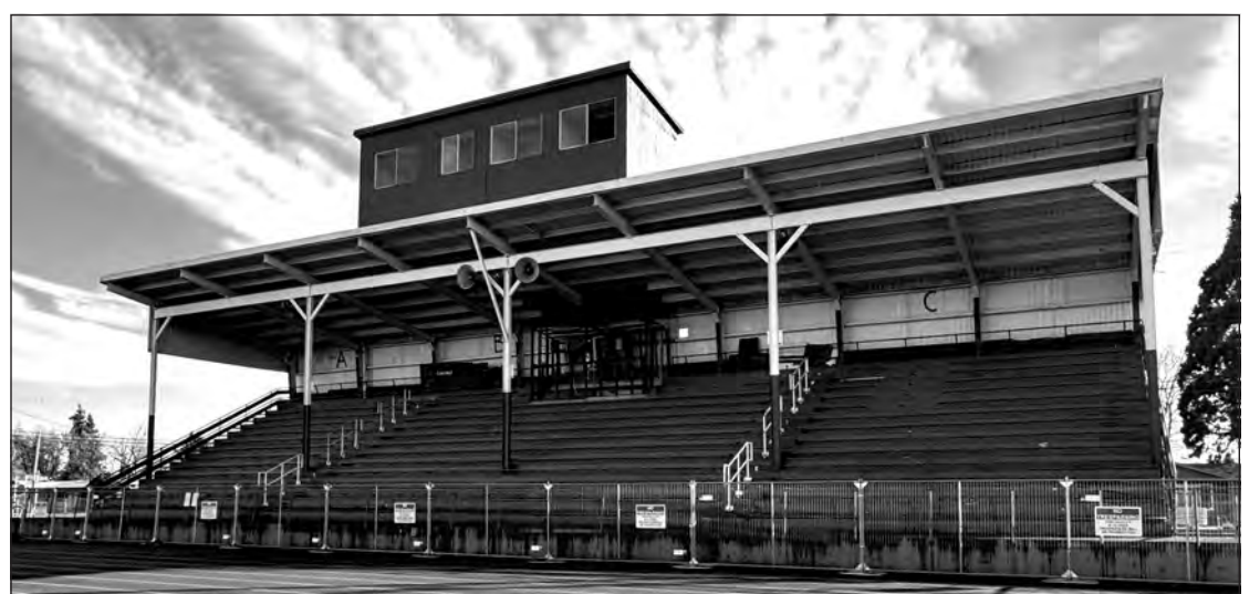
Heath Stadium prior to the beginning of demolition.
