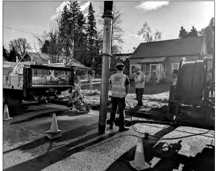
Employees with the Sweet Home Public Works Department cut through the pavement to access a water leak.
