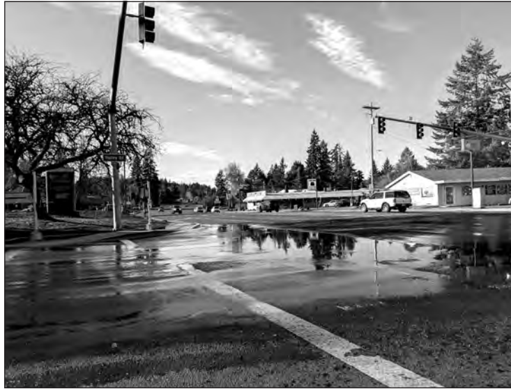
Water puddles up at the intersection of Holley Road and Highway 20 after a water main ruptured on Feb. 5.
