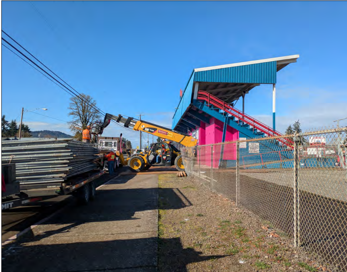
Workers begin laying down prep-work on Monday morning as the first step toward tearing down the Heath Stadium grandstand. – Photo by Sarah Brown
