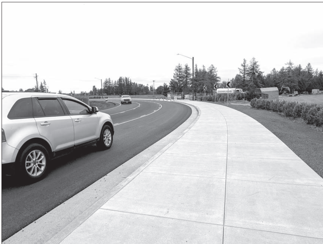
Extra wide "multi-use" sidewalks are completed along Weirich Drive at Cheadle Lake Park. Photo by Sarah Brown
