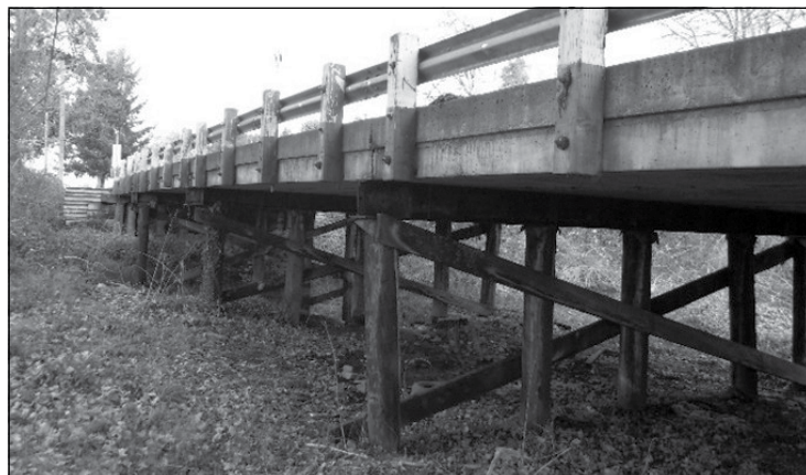
This bridge over Marks Slough is slated for repairs May 11.
