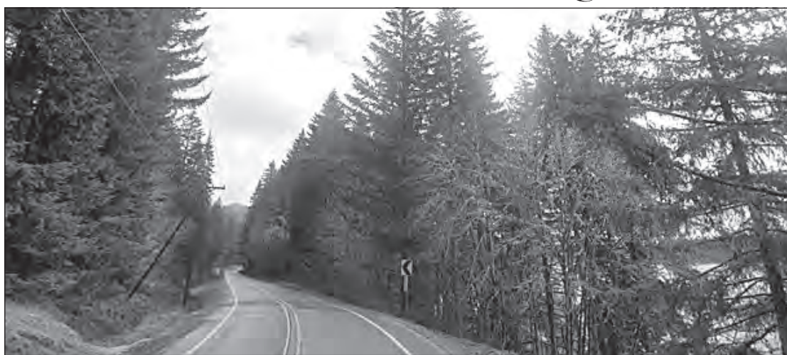
North River Drive, between Pleasant Valley and Quartzville, will undergo repairs and upgrades this summer. - Linn County photo
