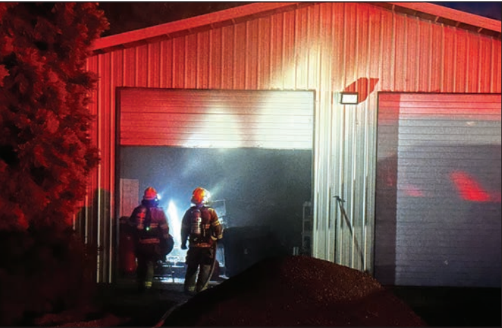
Firefighters inspect the interior of the shop, which was damaged by fire. See more photos at lebanonlocalnews.com . LFD photo
